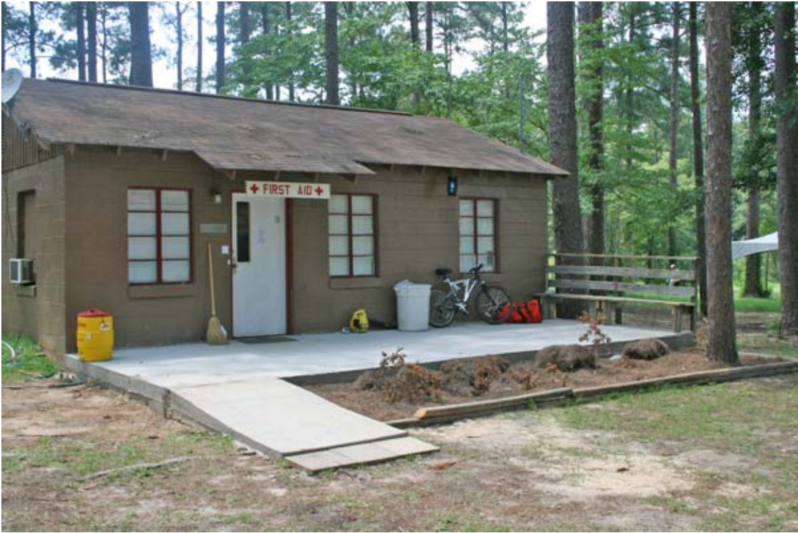
Front Porch Added to First Aid Hut
